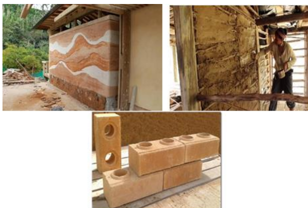
Figure 4. Ancestral techniques of wall, bahareque and compressed earth block.
